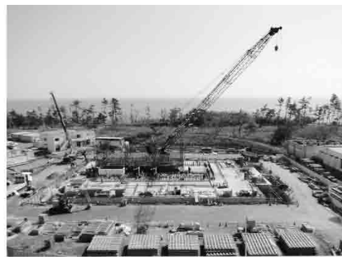
(4) The first floor (Mar. 2015)
