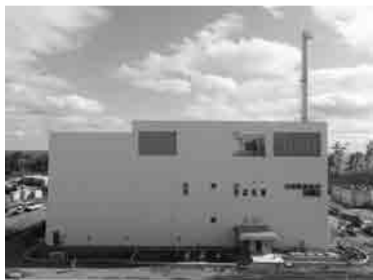
Photo 1 Construction Status of OWTF (29th January, 2018)
