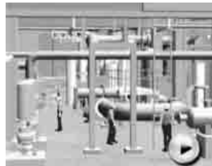
Fig. 4 Verification of reasonable dismantling procedure
