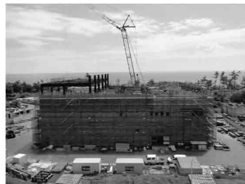
(6) The second floor (Jul. 2016)
