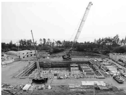
(3) The basement floor (Jul. 2014)
