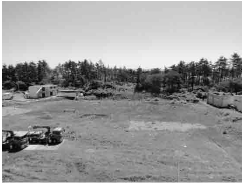
(1) Before construction (Jun. 2013)
